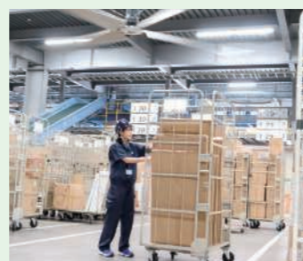
Large ceiling fan installed in the distribution center
